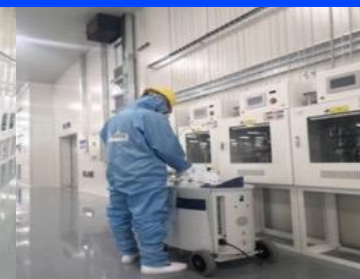
高纯管道氦测漏 Helium leak detection for high-purity pipelines
