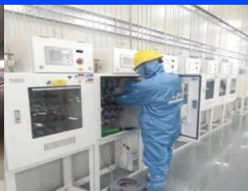
高纯管道压力测试 High-purity pipeline system connection
