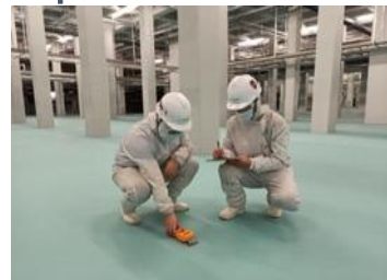
环氧地面含水率验收 Acceptance of VMB valve box materials
